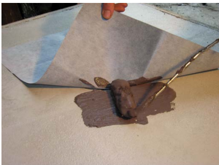
7. Apply the liquid waterproofing
