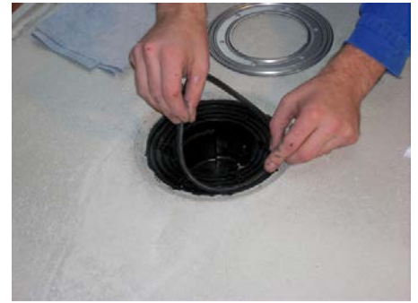
3. Remove lid cover, clean flange and insert the gasket
