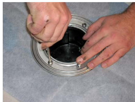
5. Fix the stainless steel ring by screwing
