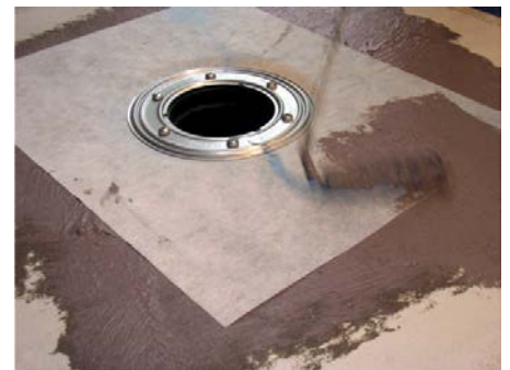
9. Apply the liquid waterproofing on the whole wet area.
