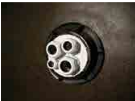
4. Insert the ready prepared pipe fairlead HL801 into the pipe sleeve HL800/160 and fix the nut of HL800
