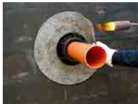
5. Weld the bitumen waterproofing
