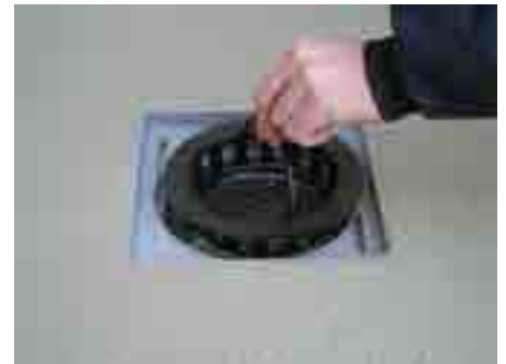
9. Remove the grate and insert the gravel catcher
