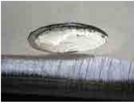
1. Create taphole with Ø 300 mm, apply prime coat, apply first bitumen layer
