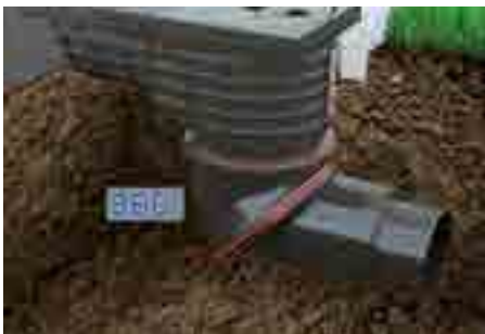
4. Adjust angle to the sewer
