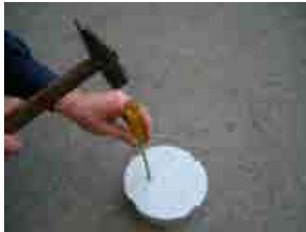
2. Select the fitting screws, depending on the quantity and the diameter of pipes/cables and open the predetermined breaking points.
