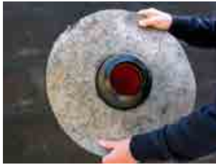
2. Set on bitumen sleeve
